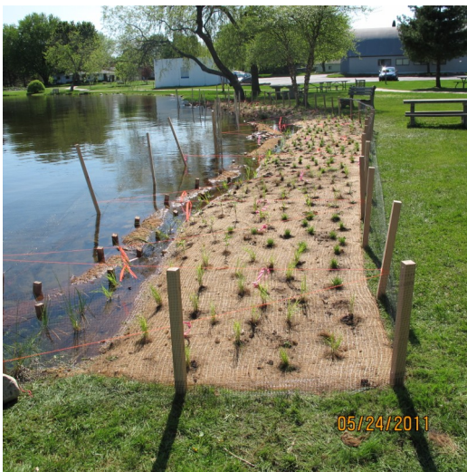
Figure 3. Newly installed 100-foot natural shoreline demonstration site at Cadillac Lakefront Park complete with temporary waterfowl exclusion fencing to protect the young plants. Photo: Jane Herbert
