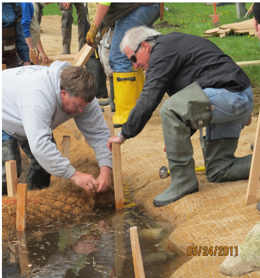
Figure 2. Contractors gain hands-on experience while installing a 100-foot natural shoreline demonstration site at Cadillac Lakefront Park during the field component of Certified Natural Shoreline Professional . Photo: Jane Herbert
